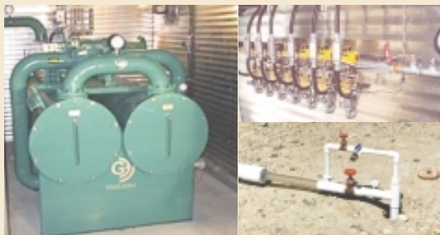
Dual Phase Vacuum Extraction with Nutrient Injector
