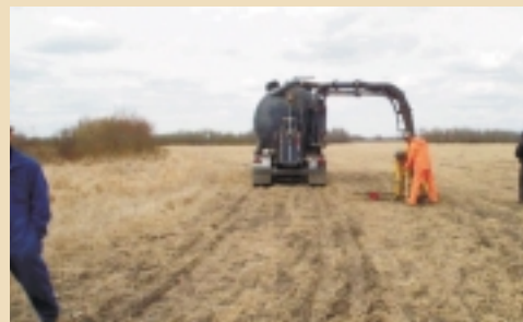
Hydro Vac of Crossing
