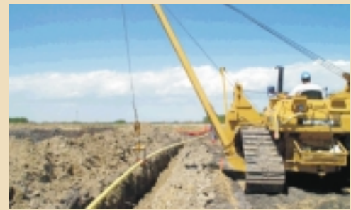
Lowering pipe into trench
