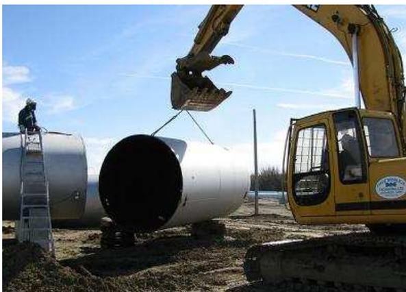
*Dismantling one of the two condensate storage bullet tanks at the Success Compressor Station.*
