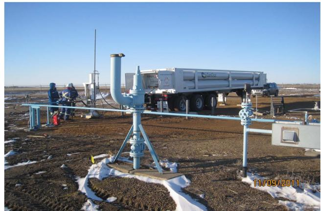
*The pilot facilities include 2" above ground piping inside the Weyburn Town Border Station, developed by TransGas, to connect to the CanGas fill post in order to load transmission line pressure gas onto transport trailers.*
