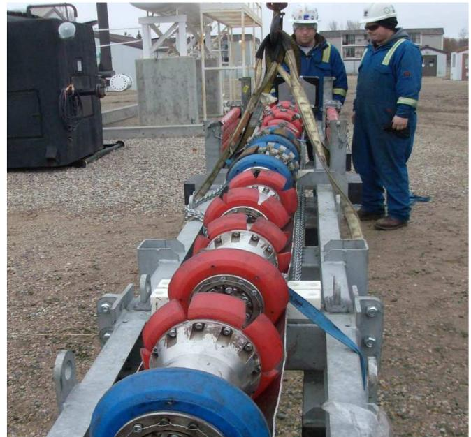
An 8" in-line inspection (ILI) tool being loaded into a pipeline.
